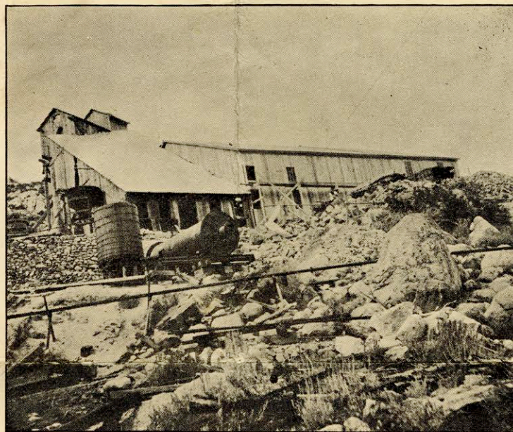
Stamp Mill House and new Cyanide House. Tube mill about ready to be rolled under the roof.
